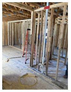
So, what did we accomplish in two days? The back bathroom and bedroom walls had been removed so that the subfloor could be replaced. The first day was spent removing the header boards where the walls used to be so that new walls could be rebuilt according to a redesigned plan. The second day was spent framing and rebuilding the new walls. Credit goes to Danny and Daniel Reed (father/ son team) who worked with Anthony who lives in the area to frame up those walls.
